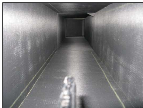
Figure 3 : View of the inside of the tested duct
