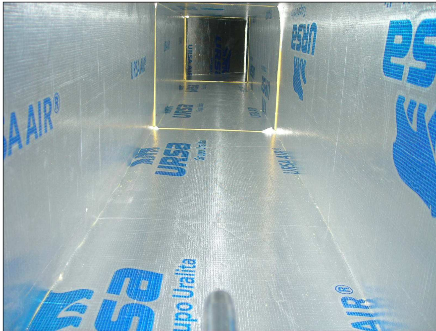
View of the inside of the tested duct
