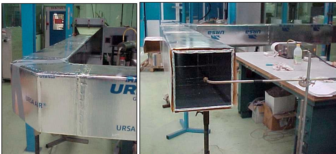
Figure 3 : Views of the installation with the tested ducts
